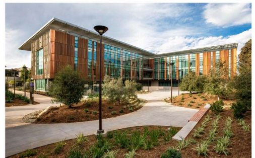
BUILDING EXTERIOR - NORTHEAST CHEN NEUROSCIENCE RESEARCH INSTITUTE
